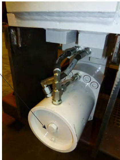
Pilot Operated Check Valve
